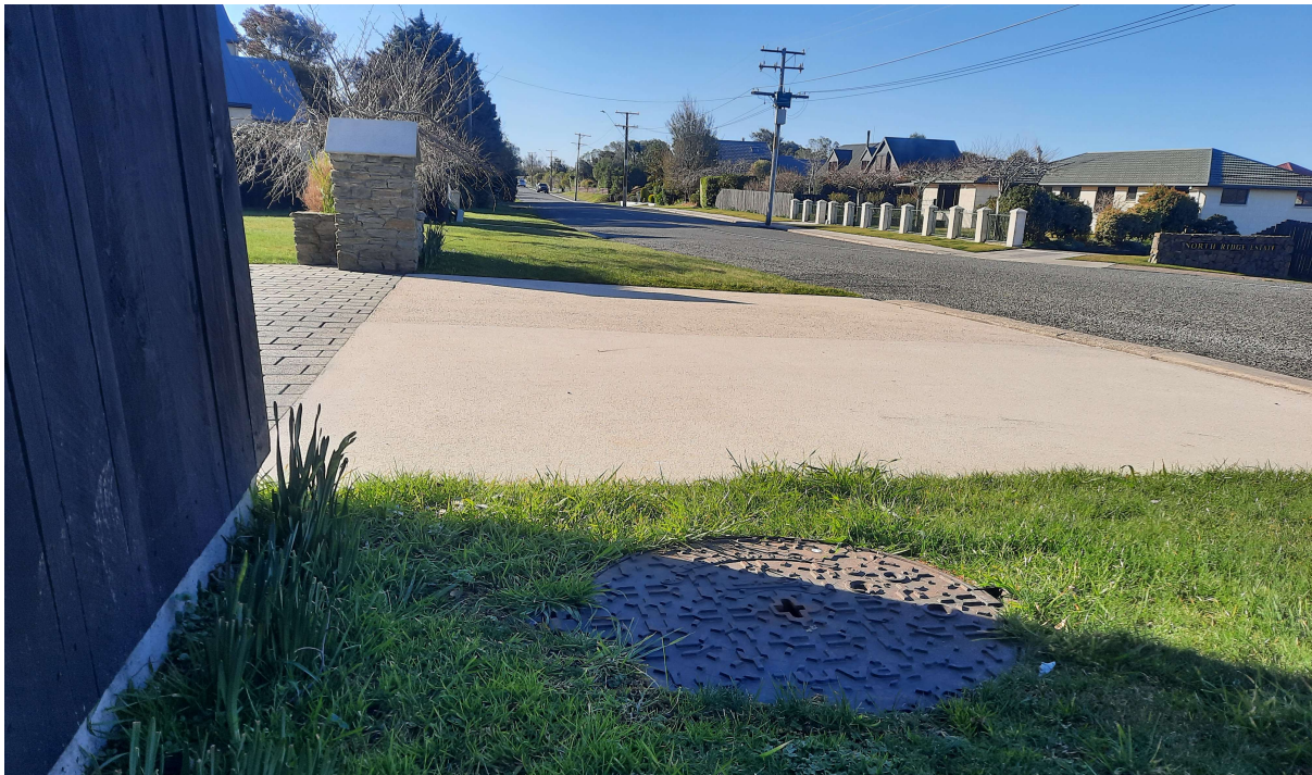
Figure 6: Existing wastewater main at a manhole near 136 Reservoir Road
