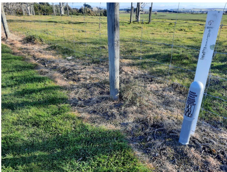
Figure 10: Existing fibre infrastructure adjacent to the site.
