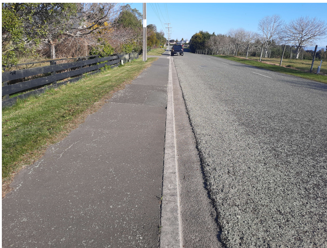
Figure 9: View south-west along Reservoir Road from the south-east side of the road.
