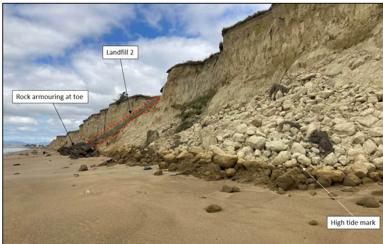
Figure 2 Cliffs adjacent to Landfill 2. High tide mark illustrated within the material accumulated at the base of the cliff.
