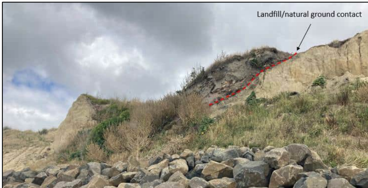
Figure 2 Northern extent of Landfill 1 illustrating contact between the landfill and natural ground
