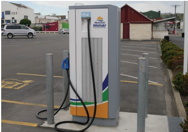
Image 32: Electric Vehicle (EV) charging infrastructure on Eden Street
