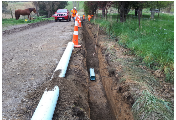
Above: Whitestone Contracting staff lay pipeline along Nuns Road, Herbert.
