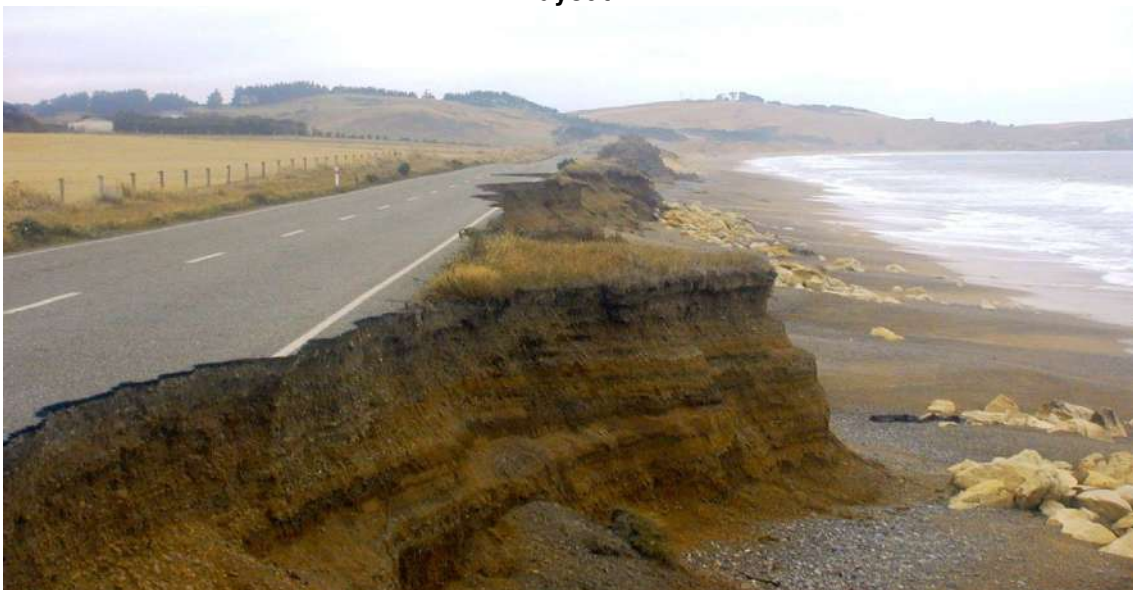
Figure 23: Site 3 – Significant damage to Beach Road
