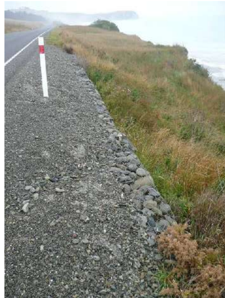
Example 2 - General view of carriageway, and shoulder protection works at a gully location
