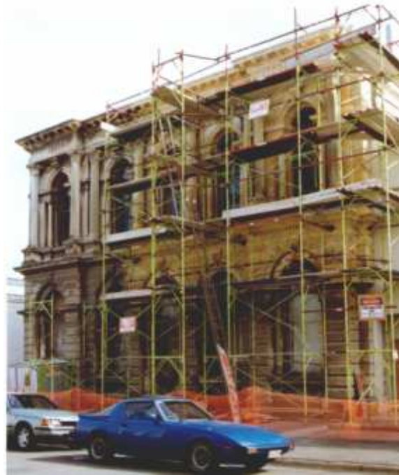
Facade cleaning underway on the former Union Bank of Australia building.
