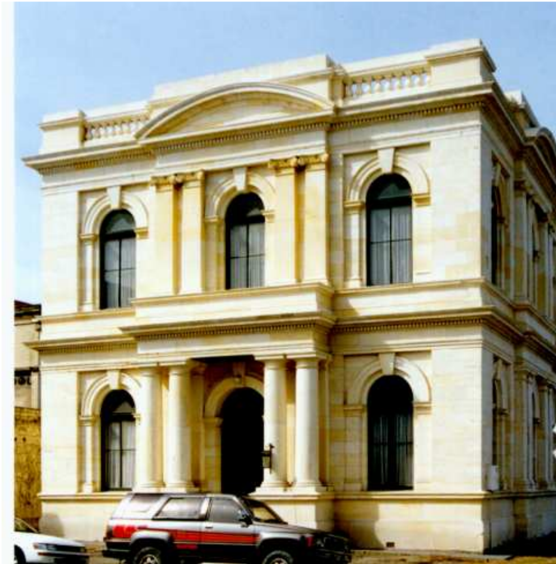
The former Customs House presents good symmetry between the two elevations. The reinstated parapet balustrade completes the original design.
