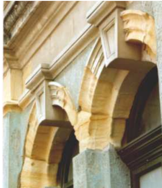
This uneven spalling of the stonework is probably caused by the stone being originally laid off its bed.
