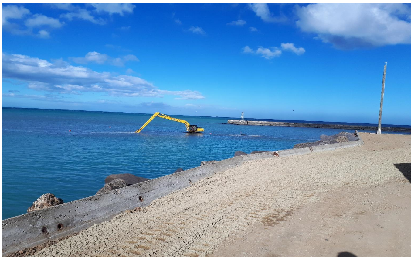
Photo showing 40 ton digger operating at northern portion of dredging area
