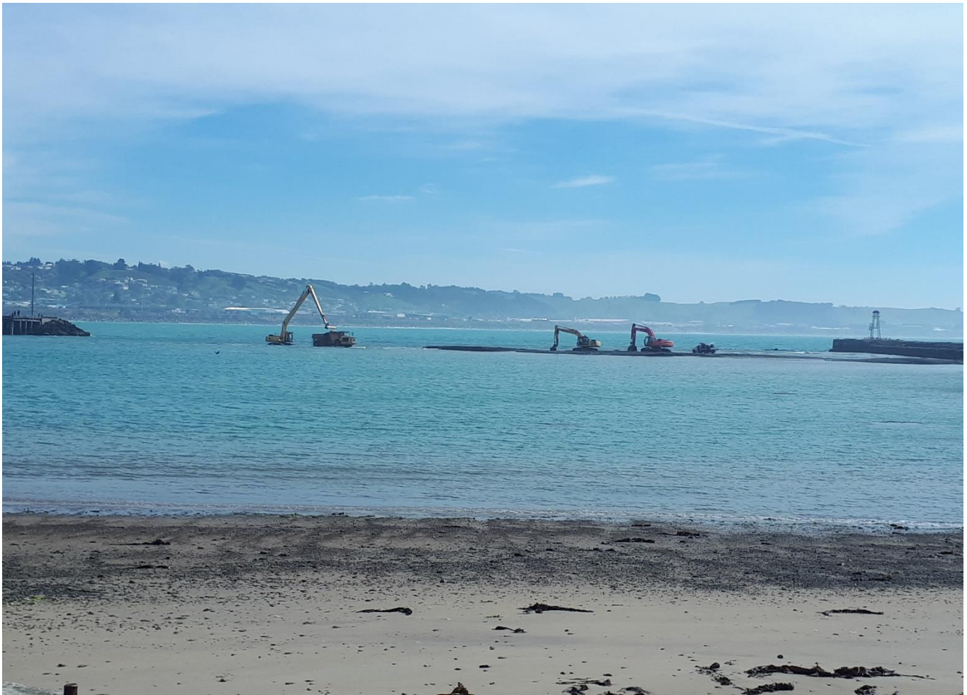
Photo taken on 24 October 2018 showing causeway formed out to the eastern edge of the dredging area
