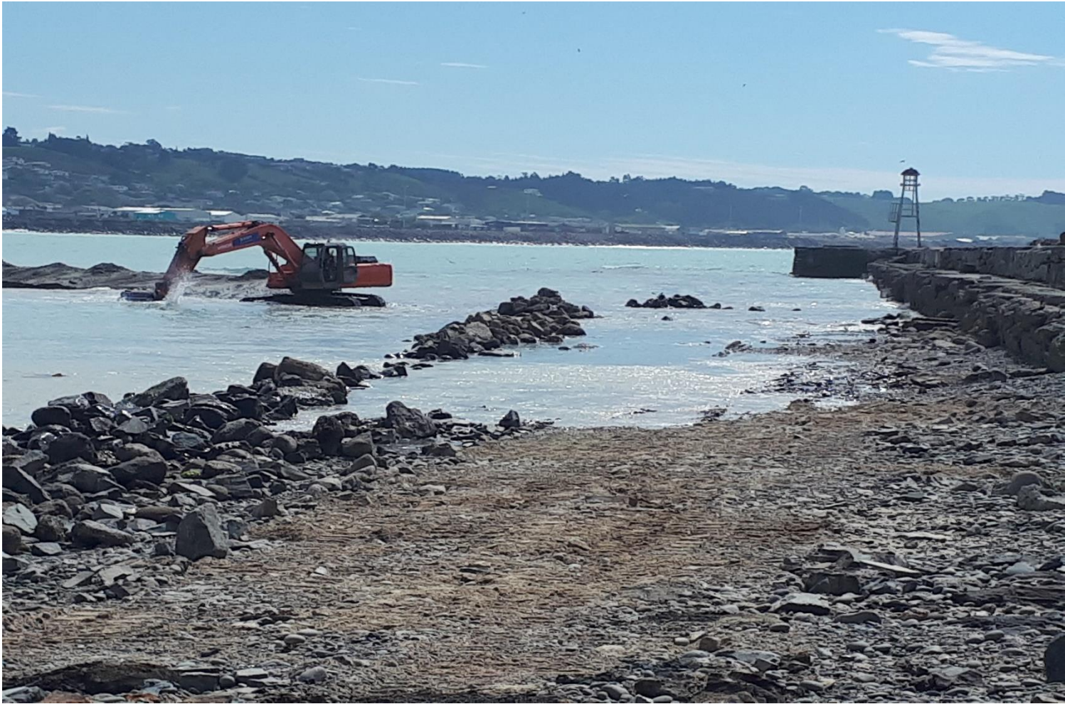
30 ton digger forming start of causeway
