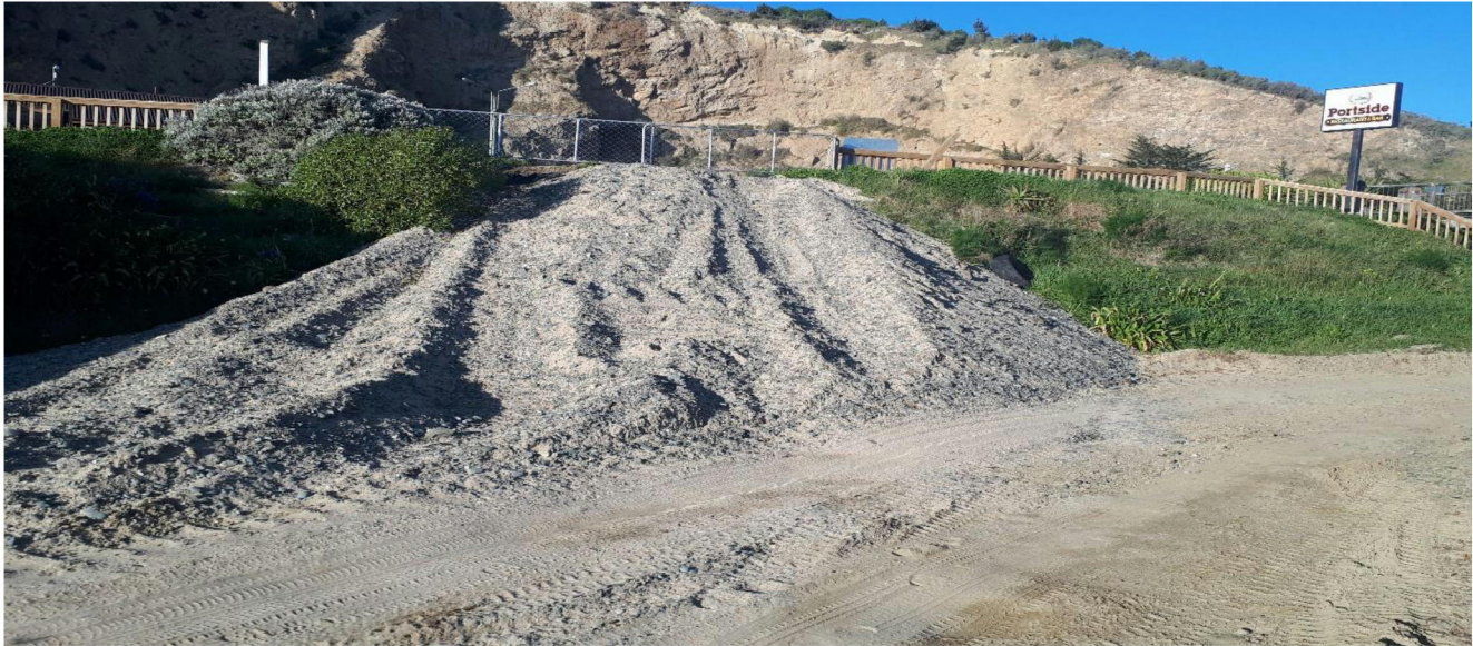
Photo of ramp formed to provide access for 40 ton long reach excavator
