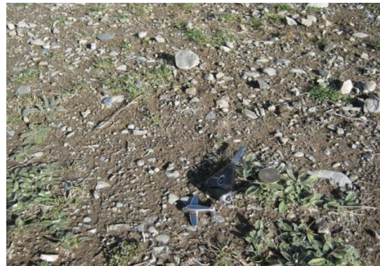
Photograph 6.2: Rock crushed existing cycle path in Mackenzie country with tight granular mosaic surface locked up with existing fine soil material.
