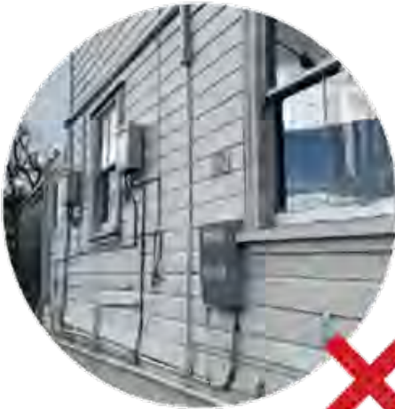
Figure A19 - Modern electrical and plumbing services including gas boiler, heatpump and connecting pipes have been added to this street facing building façade resulting in a cluttered and unattractive frontage.
