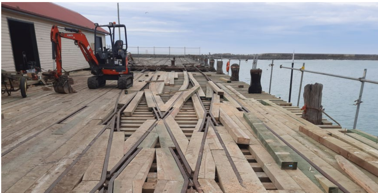
Figure 1 & 2 - Renovation of Holmes Wharf
