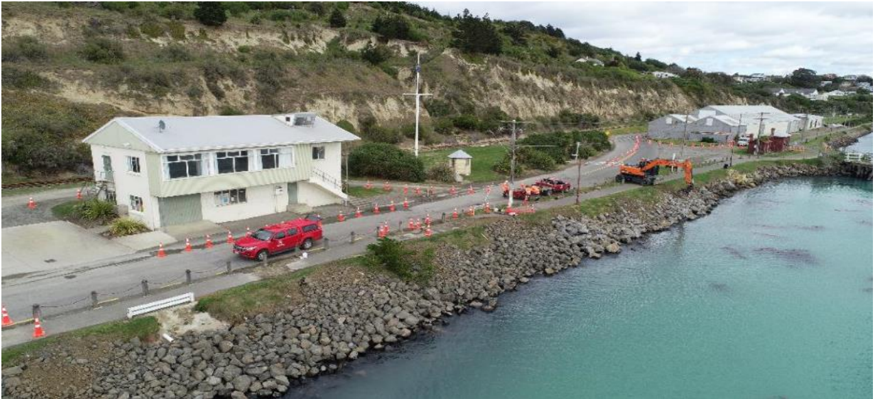
Rock revetment work at Ōamaru Harbour
