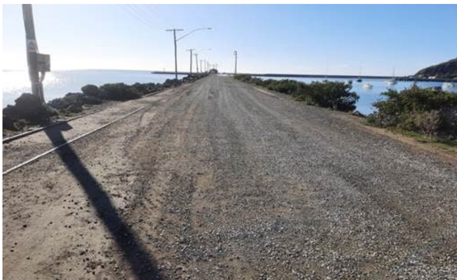
Holmes Wharf Access Road recently graded
