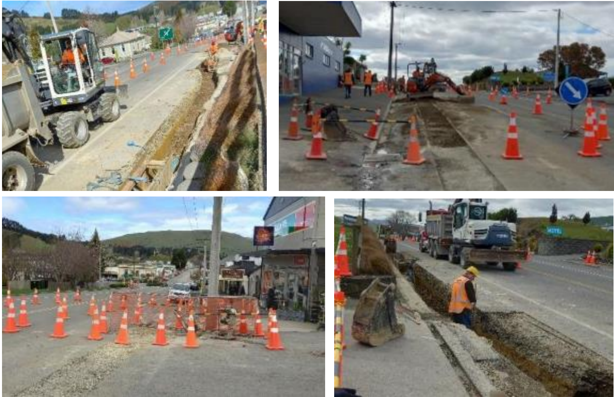
Figure 4 - Palmerston Water Mains Renewal
