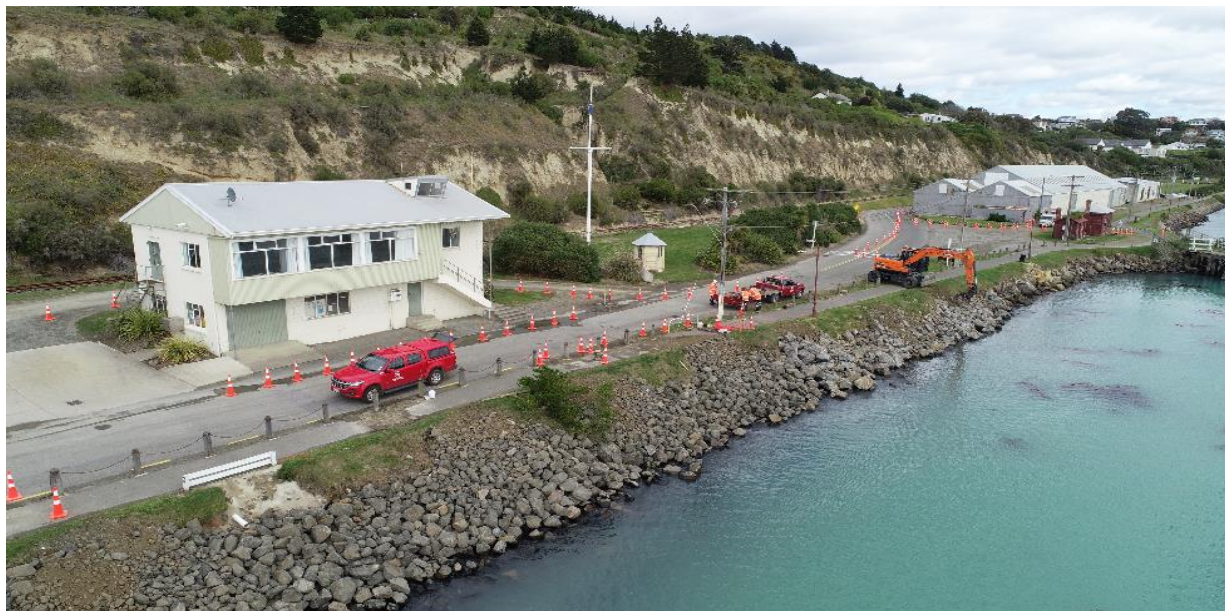
Rock revetment work at Ōamaru Harbour
