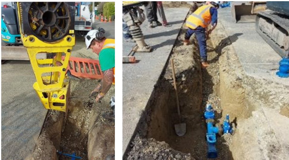
Figure 1 - Rother Street watermain installation
