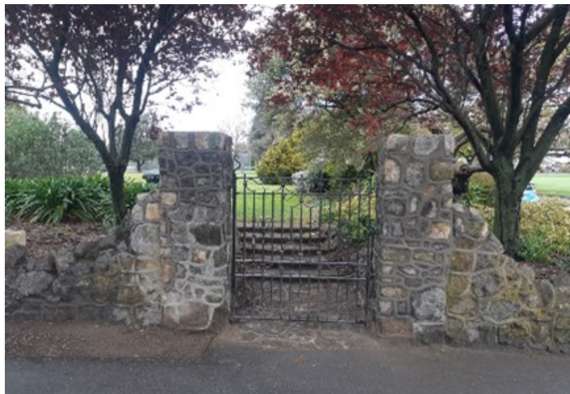
The former Awamoa Archway, now the Awamoa Pillars
