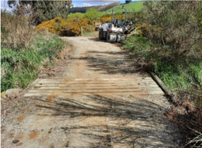
Culverts have been repaired or upgraded
