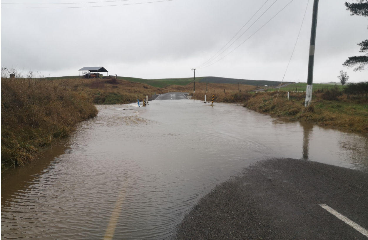
Waiareka Stream flooding
