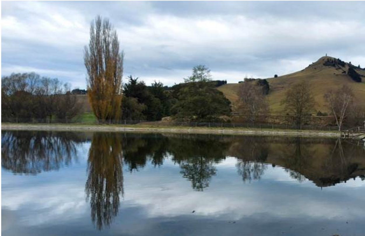
Palmerston Wastewater Treatment Plant Oxidation Ponds
