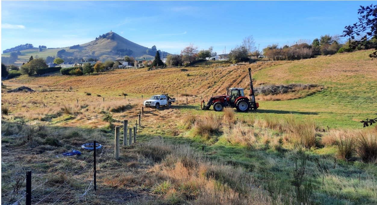
Fencing Palmerston Walkway
