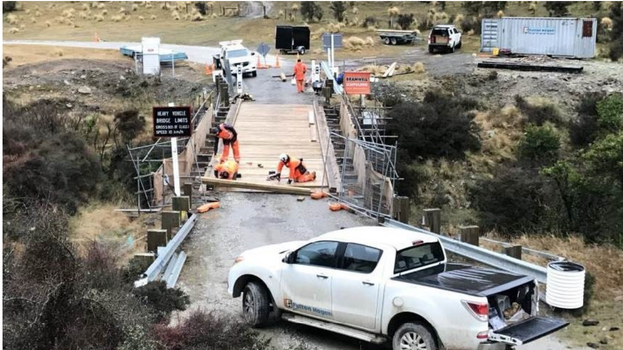
Bridge 67 Danseys Pass preparing to open with the new deck
