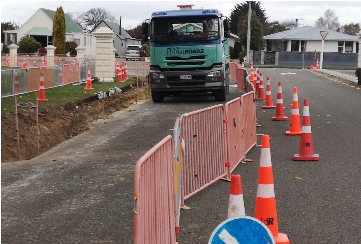
Kerb and channel renewal - Centennial Park
