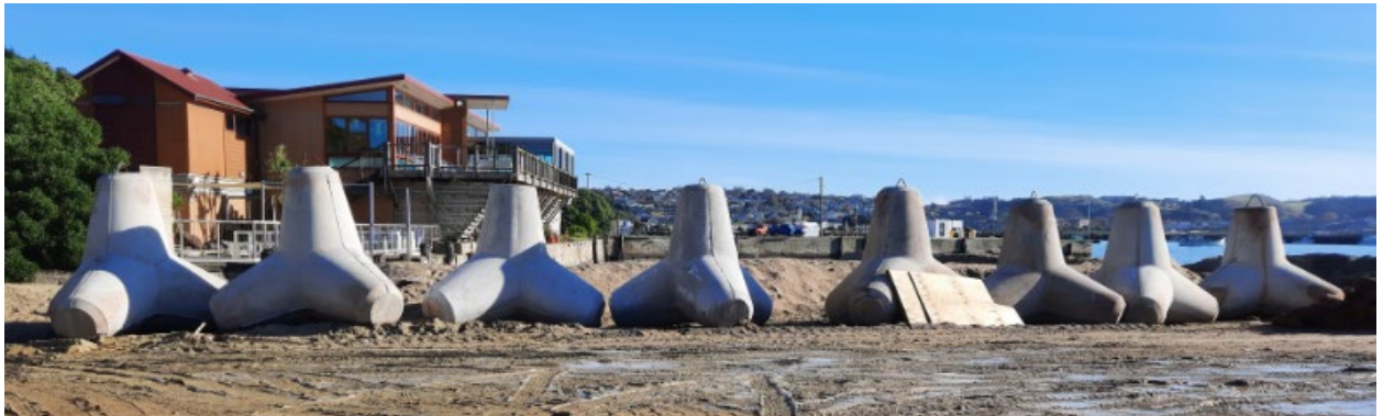
15 tonne tetrapod units ready for placement at the breakwater head
