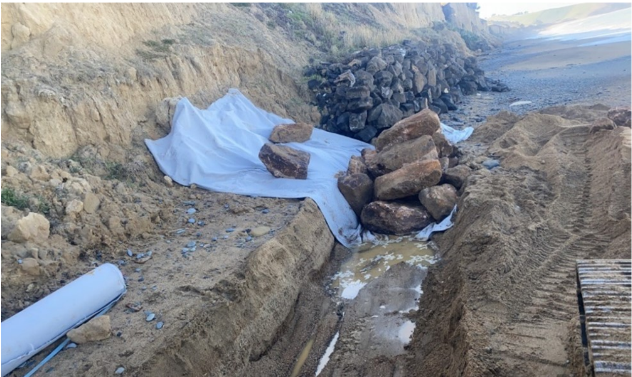
Coastal erosion repair and protection
