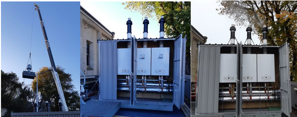
Replacement to three Baxi Luna condensing boilers (Ōamaru Opera House)
