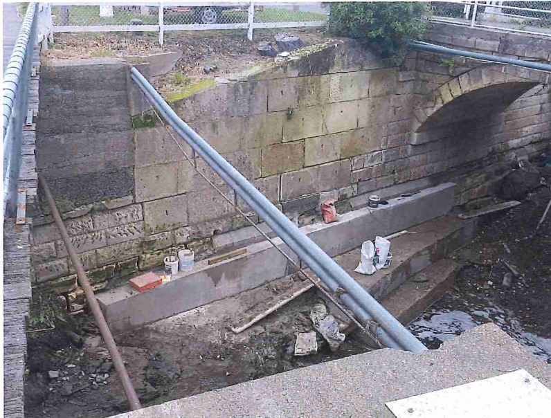
The eastern side with a solid concrete footing and a strong beam of concrete filling the main fault area
