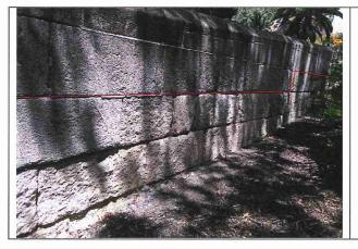
Remove top two blocks to reduce to 600mm then step up where appropriate to maintain 600mm height
