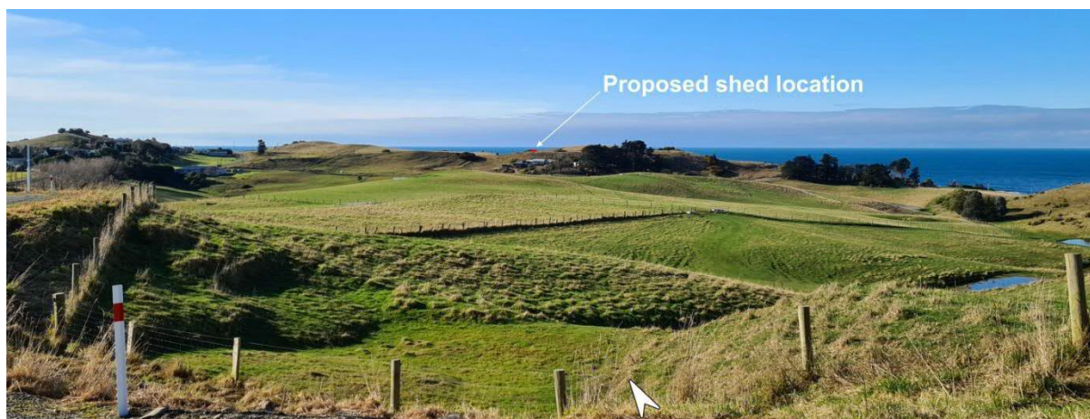
Figure 13: View from the intersection of Lighthouse Road and Kaika Road to the site at a distance of 800metres showing the proposed buildings will only be partly visible due to the upper parts of the site being screened from view by the ridgeline adjacent to Te Karita Road. The buildings will also integrate with the existing cluster of structures on the neighbouring properties.
