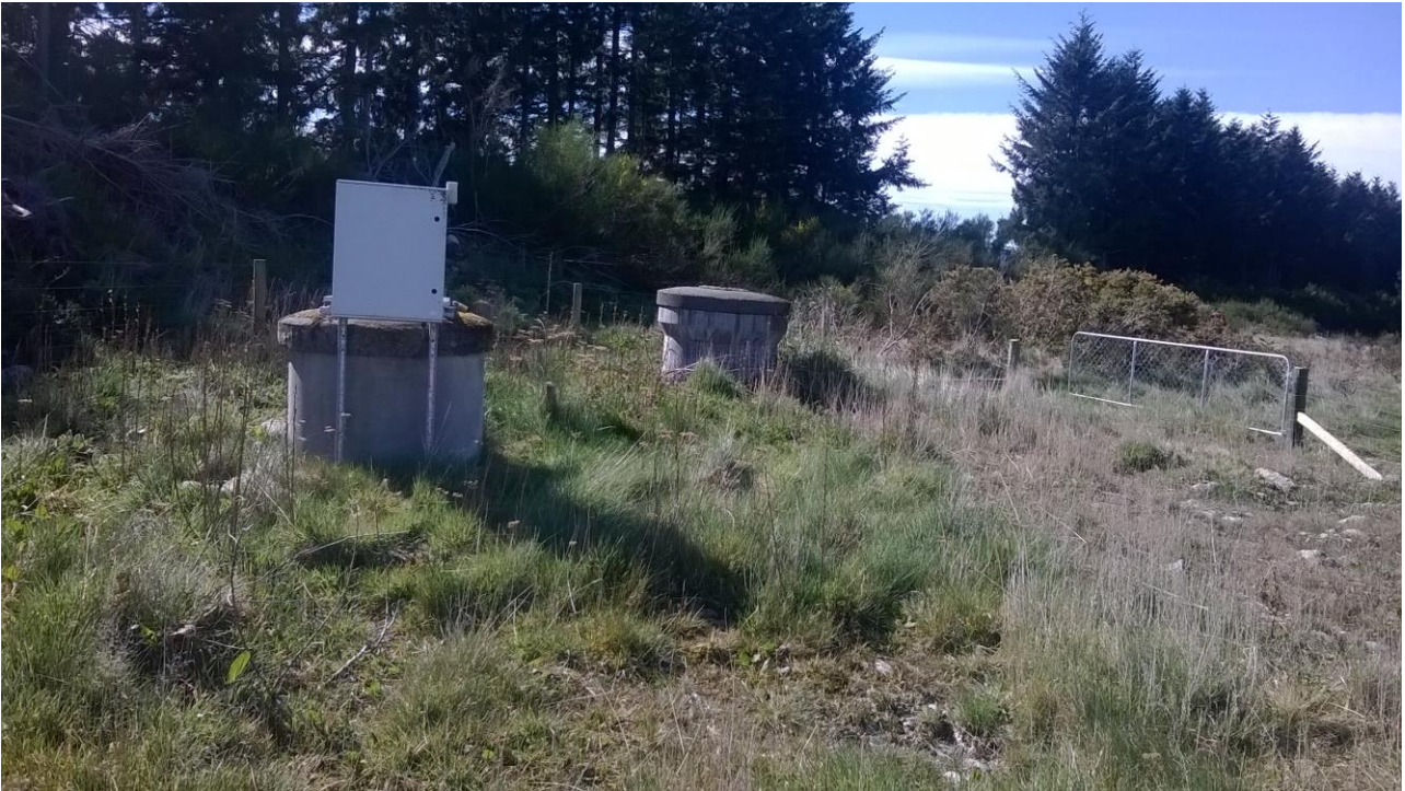
Photo 1: Intake gallery manholes inside locked compound
