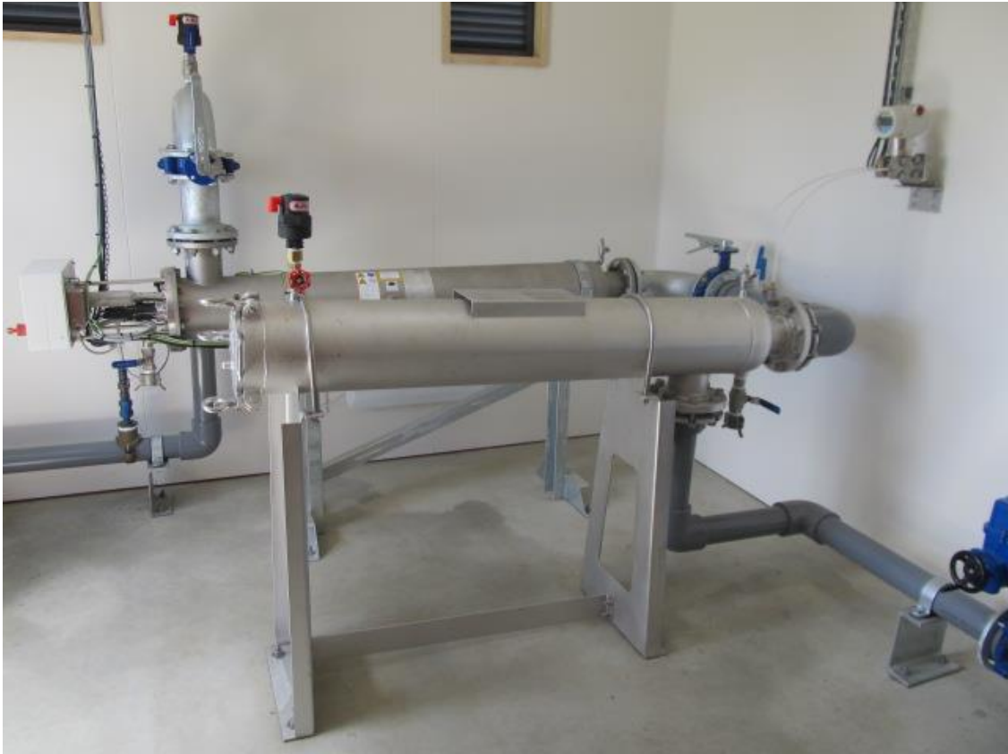
Photo 7: UV and filtration units
