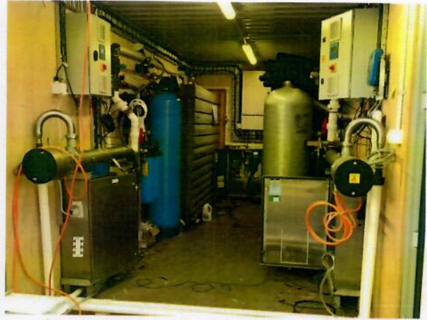
Apex containerised water treatment plant for Christchurch City Council (delivered in partnership with Citycare)
