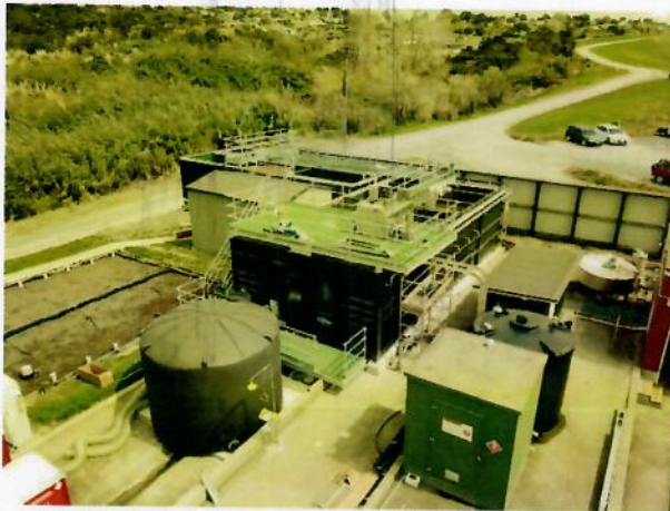
Apex containerised MBR wastewater treatment plant for Watercare (Warkworth)
