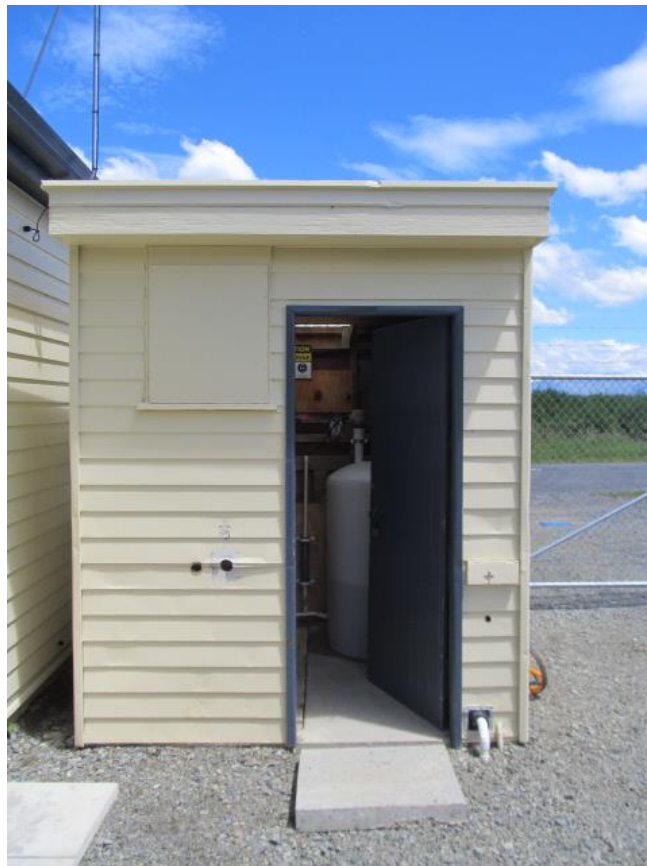
Photo 4: Chlorine dosing shed
