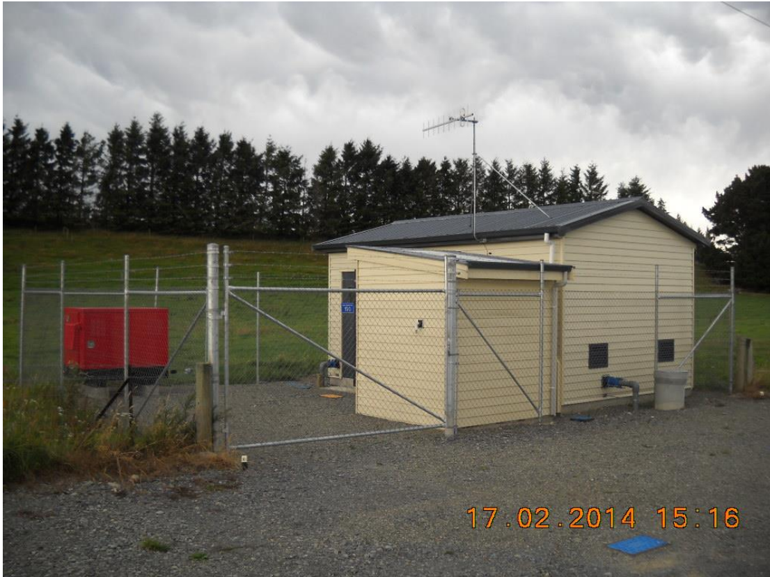
Photo 3: Treatment plant and generator
