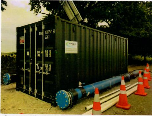
Apex containerised drinking water filtration plant for Timaru District Council
