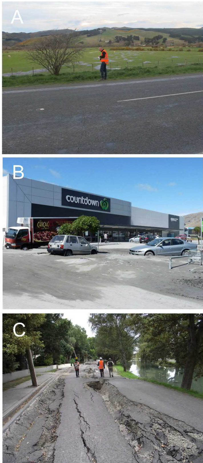
Figure 2.1 Photos illustrating some effects of liquefaction and lateral spreading. A: Relatively minor liquefaction effects in a paddock near Tai Tapu, with pods of grey sand/silt that issued from the ground during the 2010 Darfield Earthquake. GNS Science VML ID: 1398421; DJA Barrell, 5 th Sept 2010. B: Severe liquefaction effects at Ferrymead, eastern Christchurch, where vast amounts of sand/silt issued from the ground, causing localised subsidence, during the 2011 Christchurch Earthquake. EQC / GNS Science VML ID:164424; A King, 24 th Feb 2011. C: Lateral spreading and ground subsidence along a river bank in Avonside, eastern Christchurch, resulting from the 2011 Christchurch Earthquake. EQC / GNS Science VML ID: 149293; RD Beetham, 4 th March 2011.
