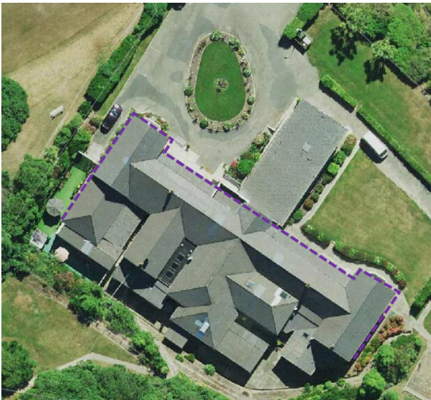
HH 22 - The Victoria Home for Aged and Incurables (Former): Extent of protection
