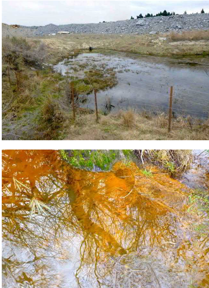
Figure 17 Top: Ponded area between the cut-off drain and haul road. Note the haul road culvert in upper centre of the photo. Bottom: Flocs of iron-staining bacteria over filamentous algae in the Camp Creek tributary downstream of Horse Flat Road.
