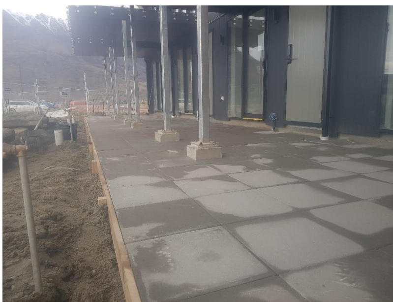
Paving work Remarkables residences 2020
