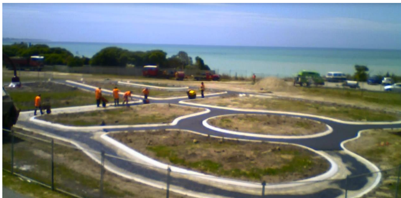
Oamaru Bike Skills park during construction
