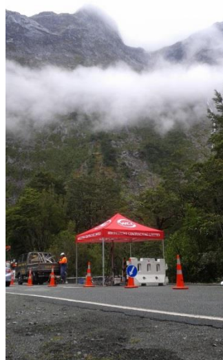
Milford Sound Bridge repairs 2016
