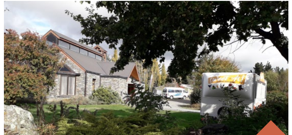
iSite building along SH8
