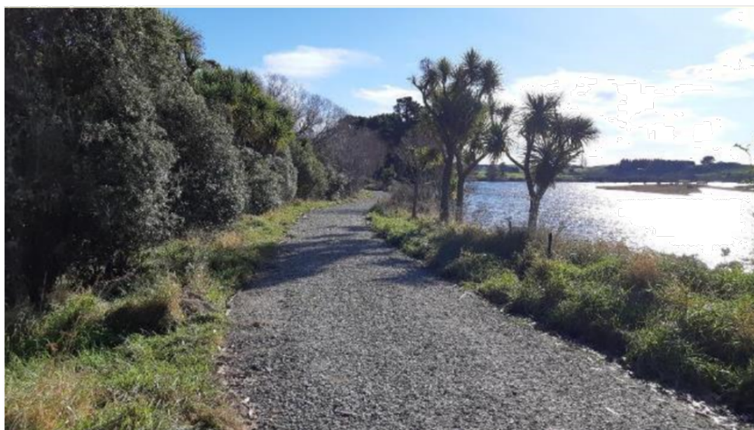
Figure 7 River Road, completed works
