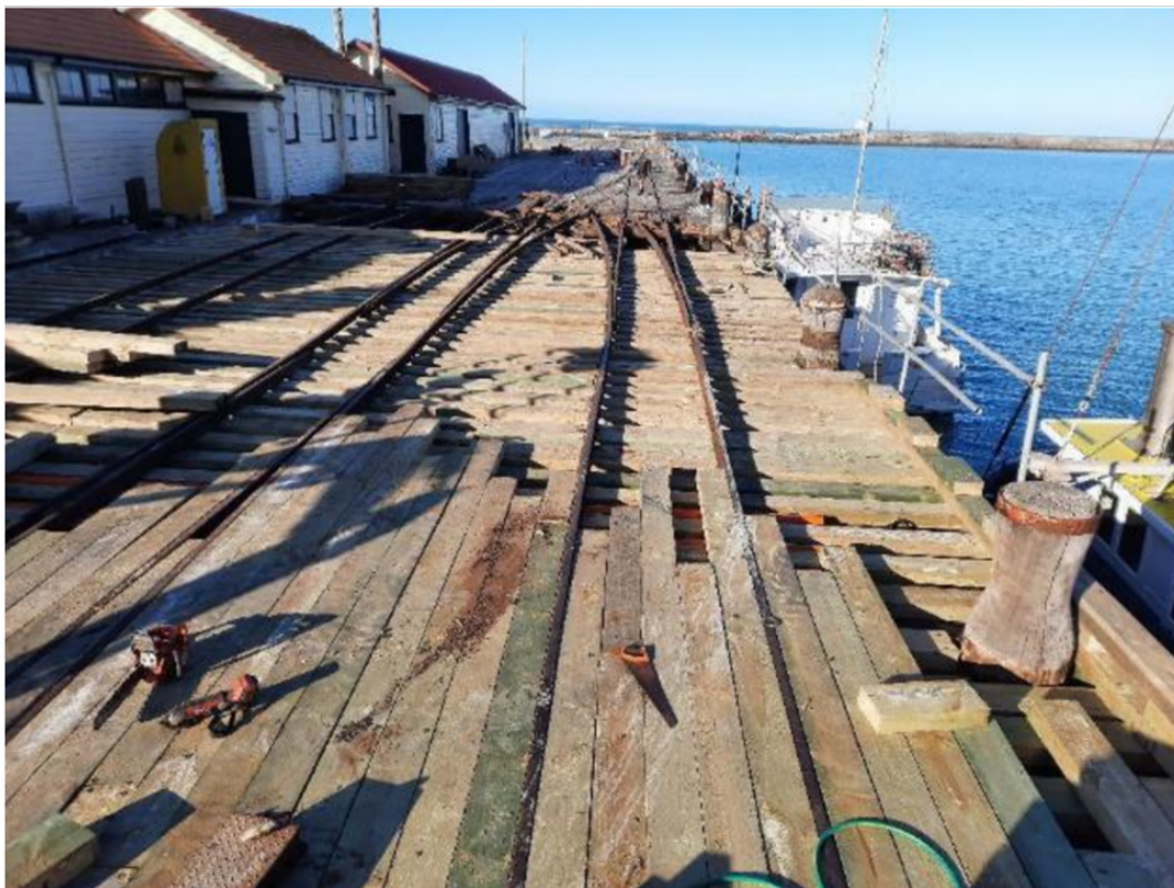
Figure 17 Decking replacement on Holmes Wharf
