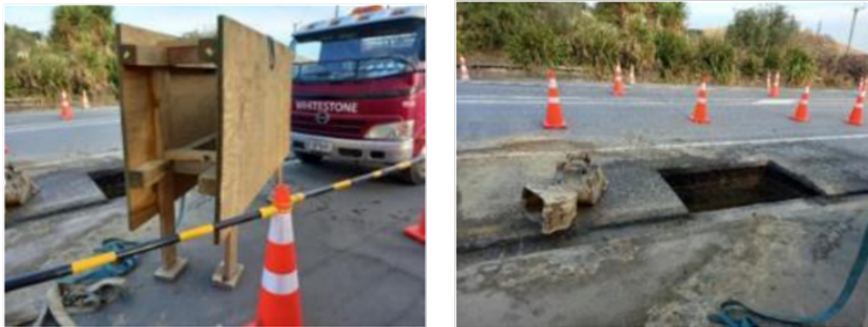
Figures 5 and 6 – Trench shield and excavation for hydrant installation
