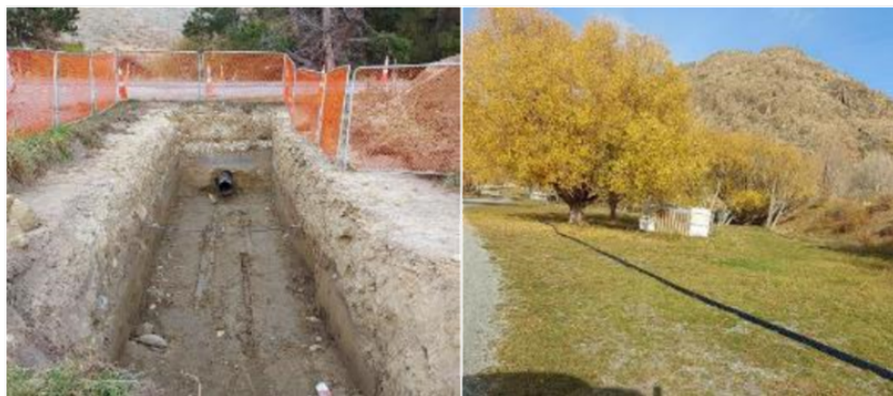
Figure 2 Parsons Rock state highway crossing and Figure 3 New PE watermain pipe prior to being installed through campground
