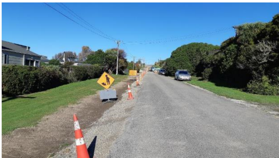
Figure 8 Kakanui Stormwater Project, Stage One Stirling Street
