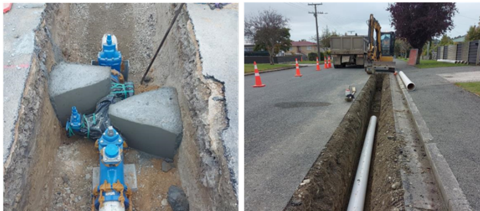
Figures 3 & 4 - New valves, fire hydrant and watermain installed on Charles Street
