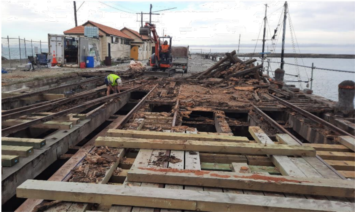
Figure 19 – Decking replacement on Holmes Wharf
