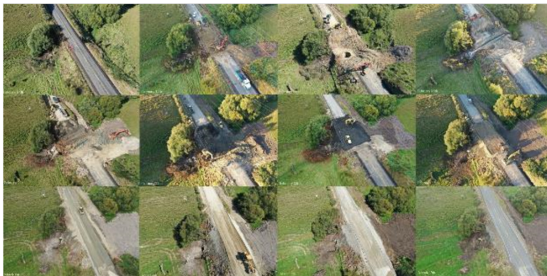
Figure 5 Airedale Road sinkhole montage
