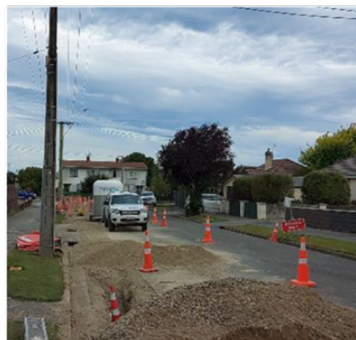
Figures 1 & 2 - Old valve removed from Dacre Street and new watermain installation on Dacre Street
