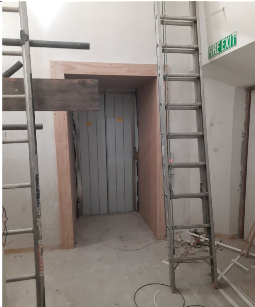
The lift installed in the museum
