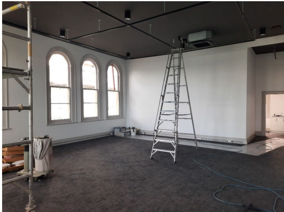
Upstairs temporary exhibition space with carpet and lighting track installed
