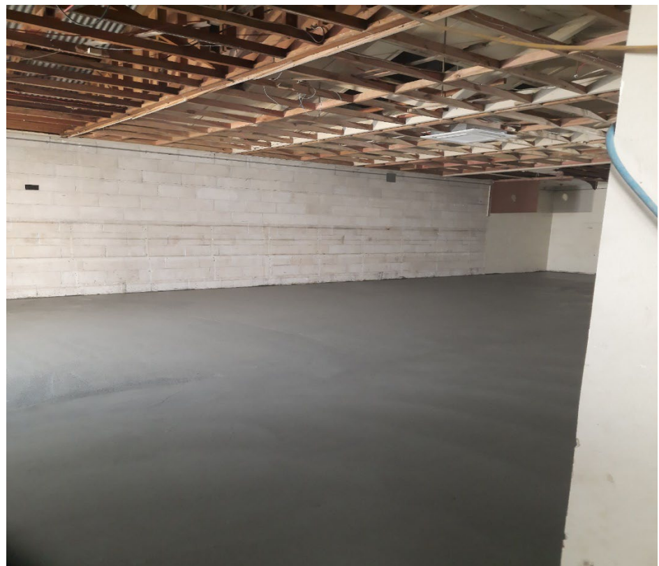
The new concrete floor in the museum storeroom
