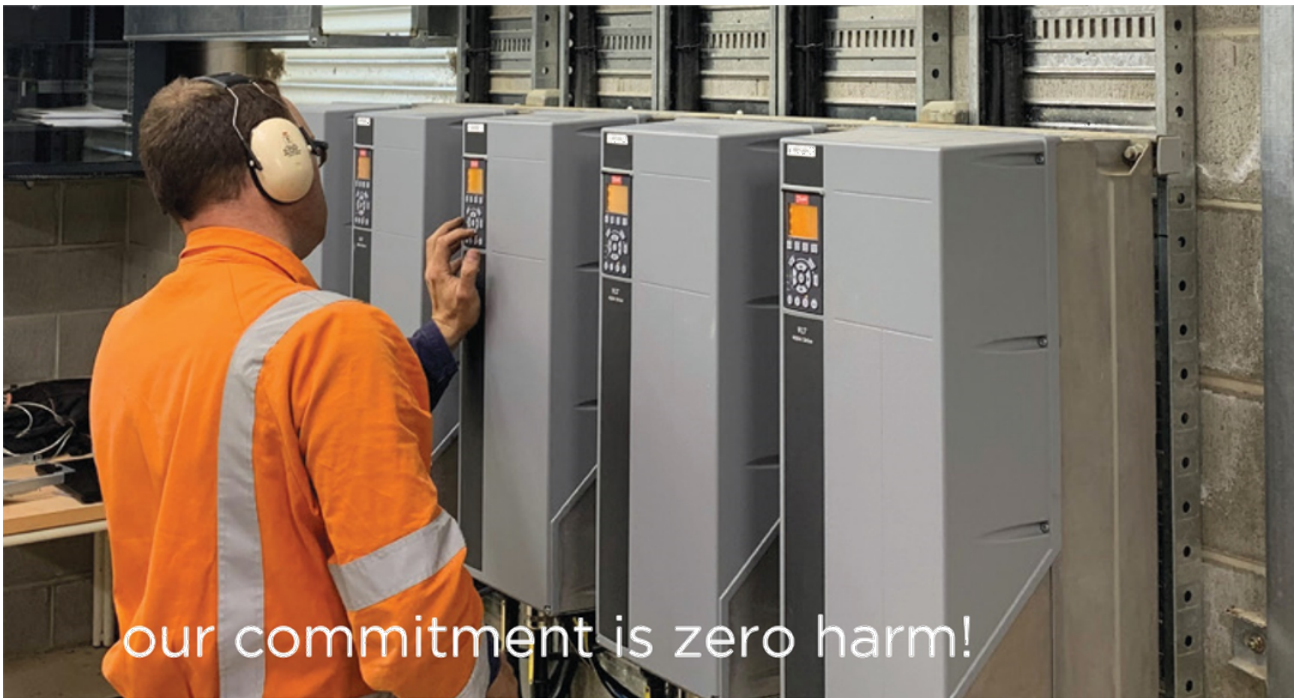
Ian Richards, drive technician of DRS, servicing variable speed drive (VSD) units at Glen Settlement extension pump station
