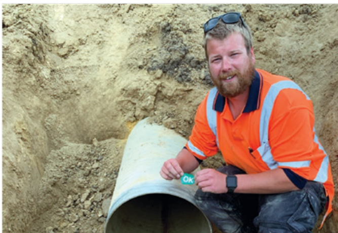
NOIC operator Will Fisher giving a newly-installed underground supply pipe the all-okay
