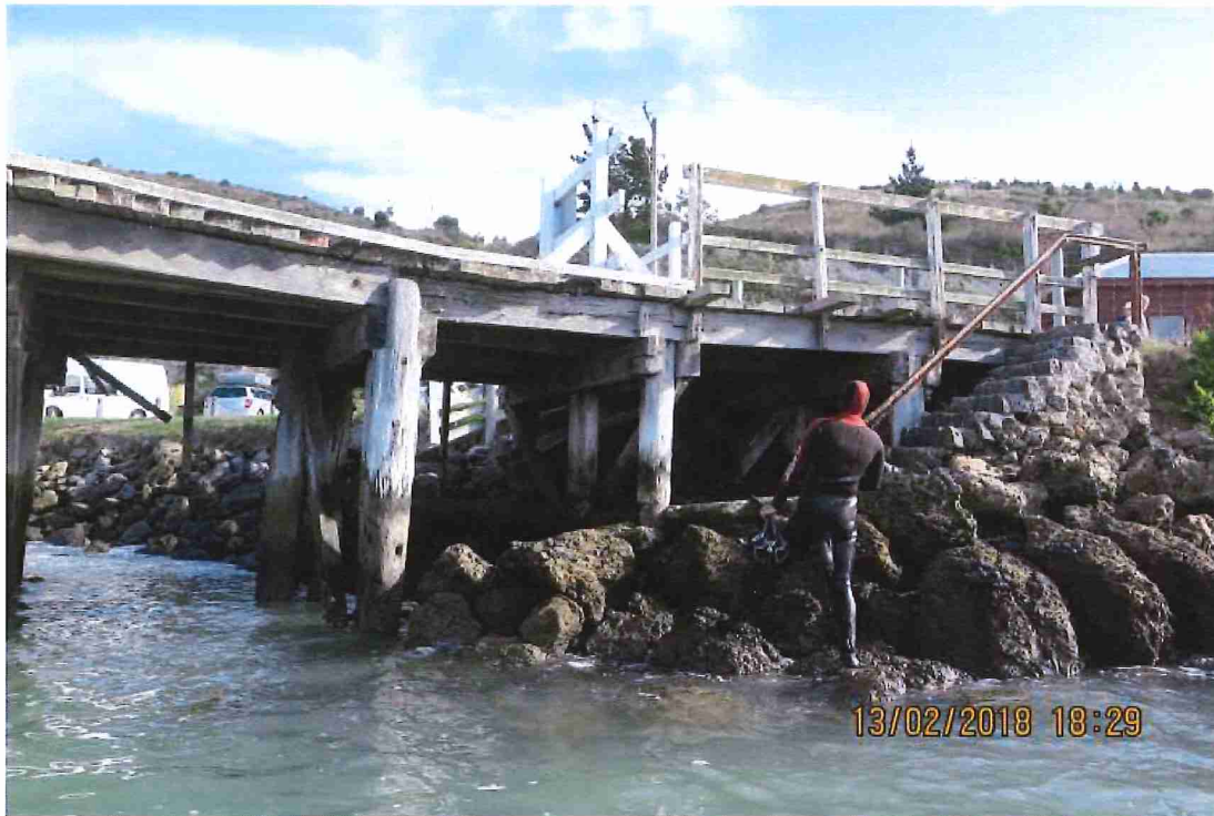
Photograph No 1: Pile bents 1 – 3 (from right to left). White barrier fence above bent 2
