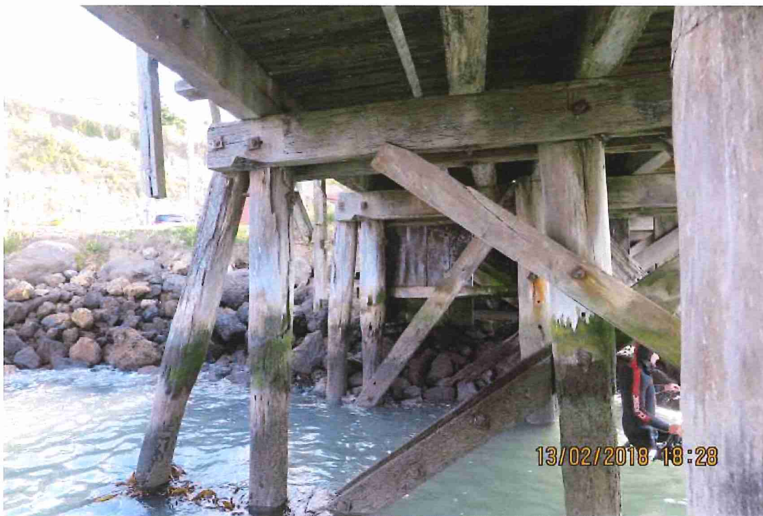
Photograph No 4: Bent 4 (foreground), bent 3 (background)
