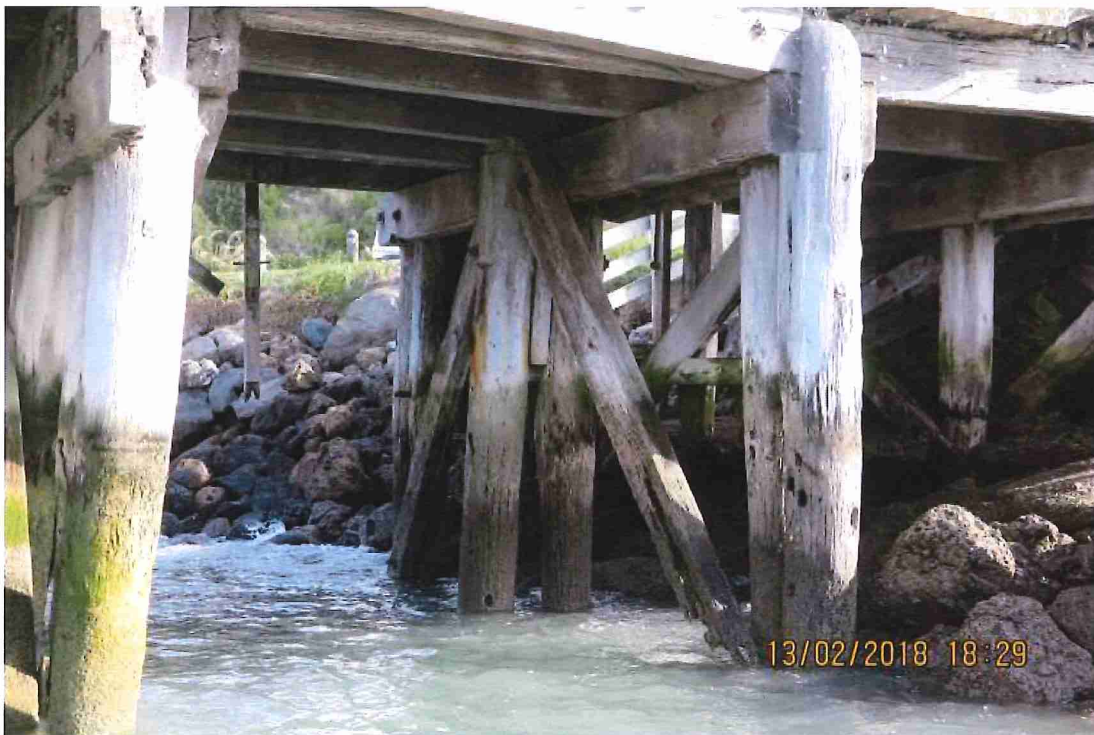
Photograph No 2: Pile bent 3
