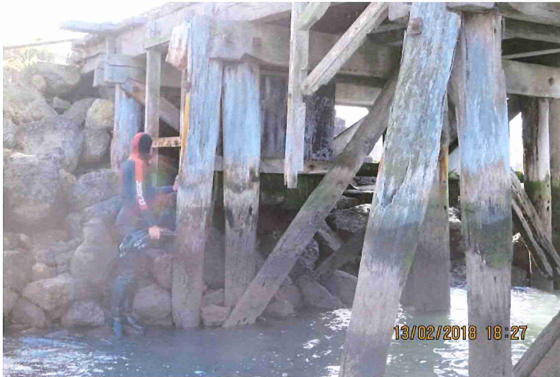
Photograph No 3: Heavily waisted load bearing pile second from left - pile bent 3
